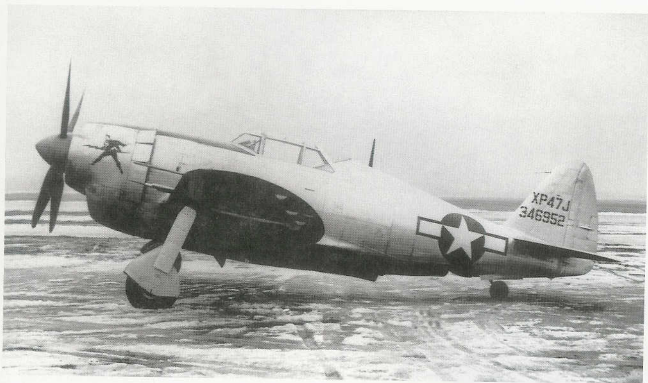
Above: The XP-47J was a project to evaluate the fan-cooled R-2800-61 engine. Initial plans called for an Aeroproducts counter-rotating propeller, but a standard four-blade propeller was fitted. The XP-47J program was ended in favor of the XP-72 covered below. The art on the cowling is an early rendition of Superman. (USAFM)
