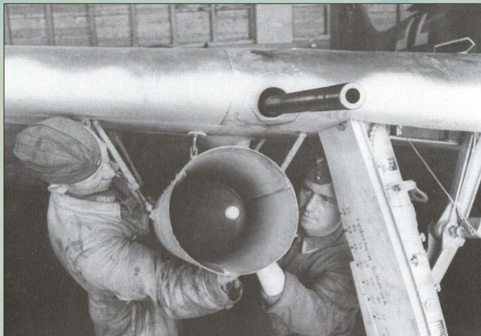
Installation of 21 cm rockets into their launchers under wings of a Fw 190A. (Bundesarchiv, archiv Eduard, www.deutschlufwaffe.de )
