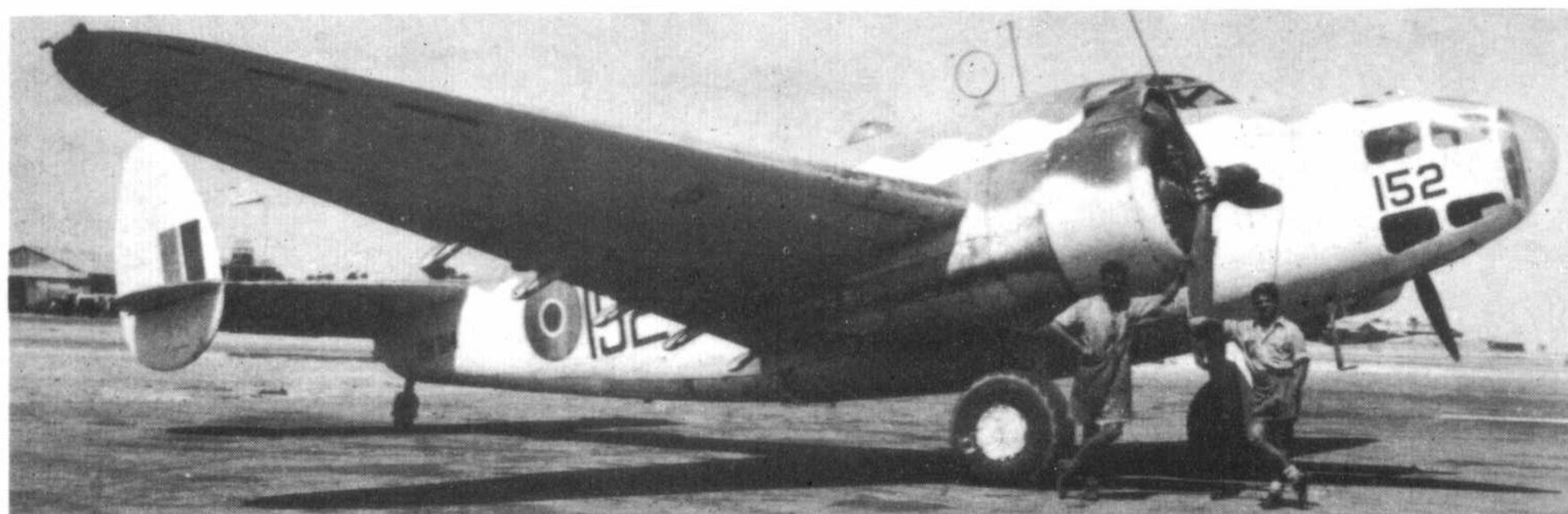
A-for-America and Lend-Lease; a Mark IIIA (FH314) at Fayid in Egypt, 1944. For local operating conditions, extra-large, Martin Baltimore-type, scoops replace the normal carburettor intakes on top of the cowlings. Exhaust flame-damper extensions are in evidence. (Photo: via Air-Britain)
