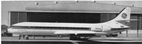
The first fan-engined Caravelle (c/n. 42) shown (above right) in original Series III form as F-WJAM, and (below) after re-registration as N420GE and re-engining with CJ805-23C's by General Electric.
